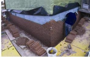
In typical installations, it allows workers to stand on the lower outrigger planks and to have material handy, on either the top outrigger planks or the platform deck. This concept will minimize risk of back injuries while providing a productive work area.
